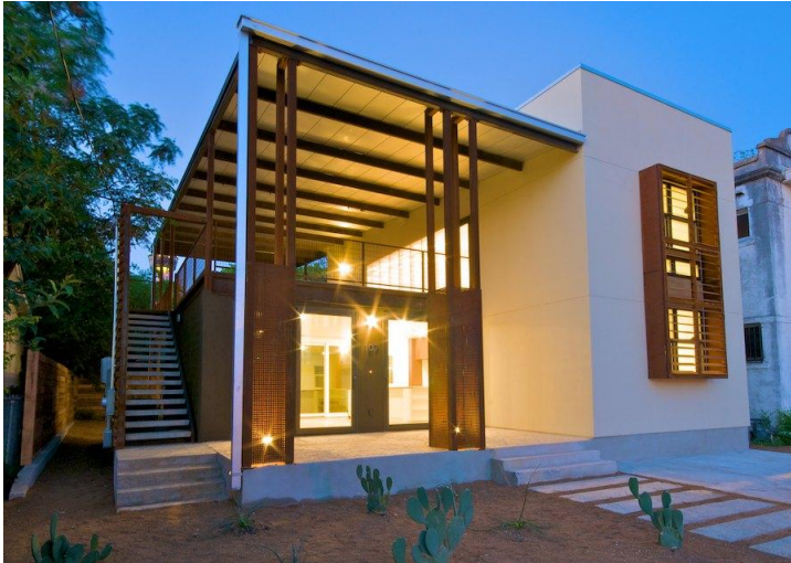
CVF Homes project at 107 Leigh Street The solar PV system is on the roof above the second-story outdoor living area
