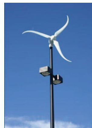
Skystream 1.8kW turbine dual-use on lamppost
