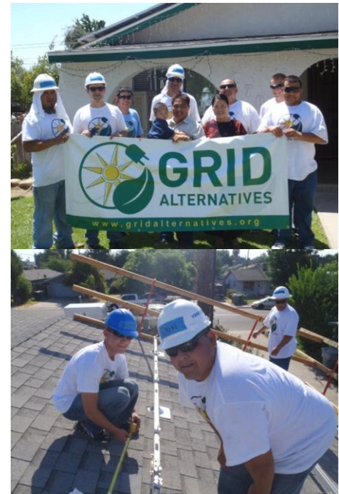
GRID Alternatives solar installation in Visalia
