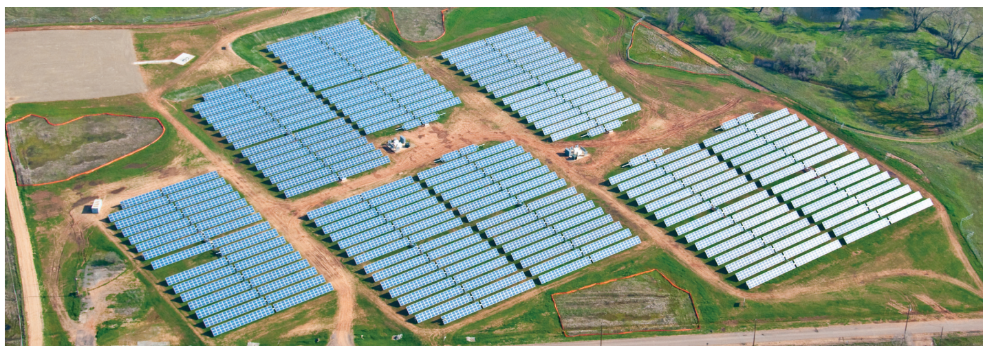
Aerial view of the Aerojet solar farm, 2009
