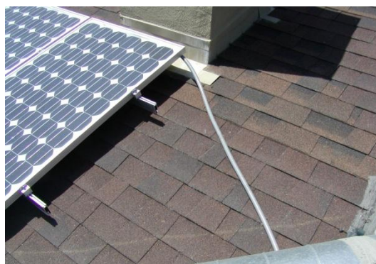
Figure 5 (incorrect) NMFC without support
