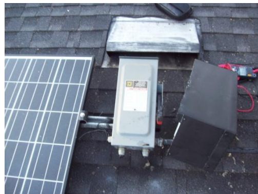
Figure 13 incorrect NEMA 3R disconnect on sloped roof designed for vertical mounting only
