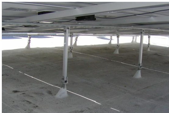
Figure 14 properly flashed roof penetration (correct)
