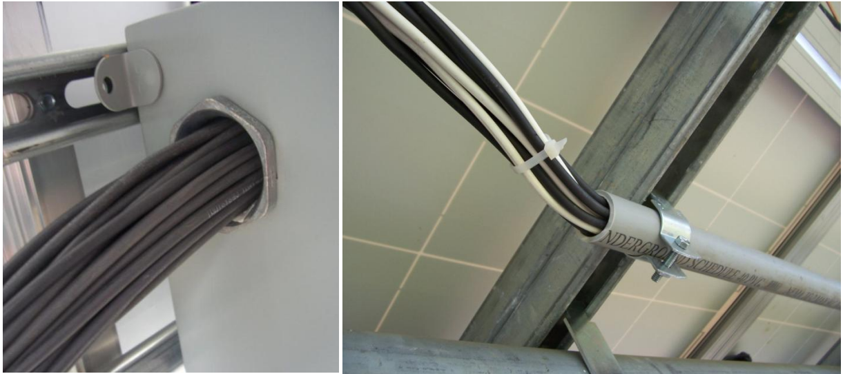
Figure 11 improper use of chase nipple and exceeding conduit fill with no end fitting (incorrect)
