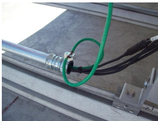
Figure 4 conductors properly protected by raceway with grounding bushing (correct)-should be secured within 12 inches of fitting (not shown)
