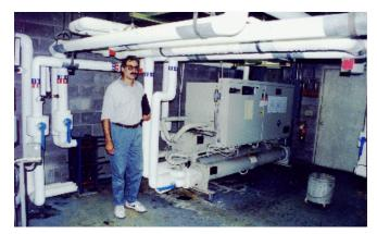
Figure 3. City Hall geothermal heat pump.
