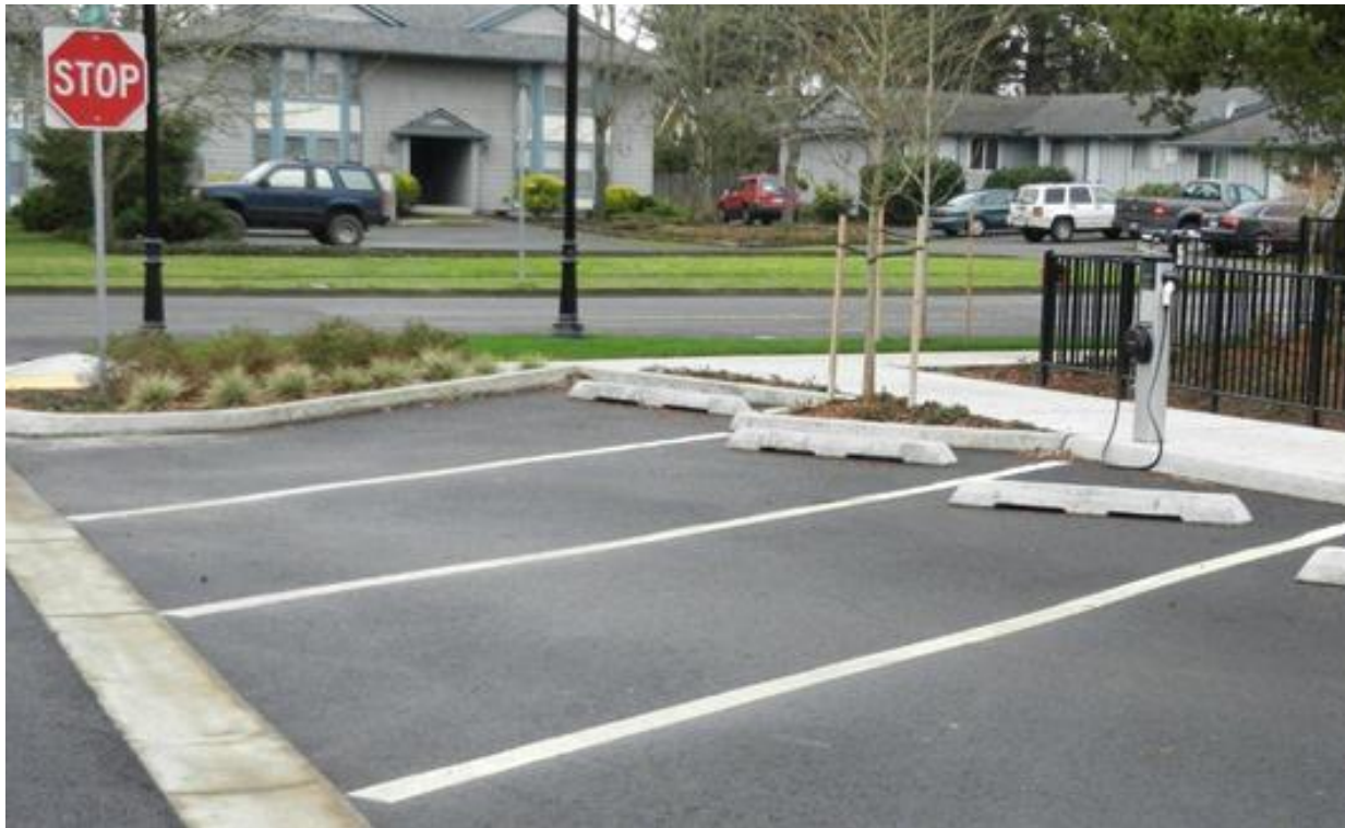
FIGURE 8: LEVEL 2 EV CHARGING STATION AT ANGLED PARKING IN RIGHT-OF-WAY
