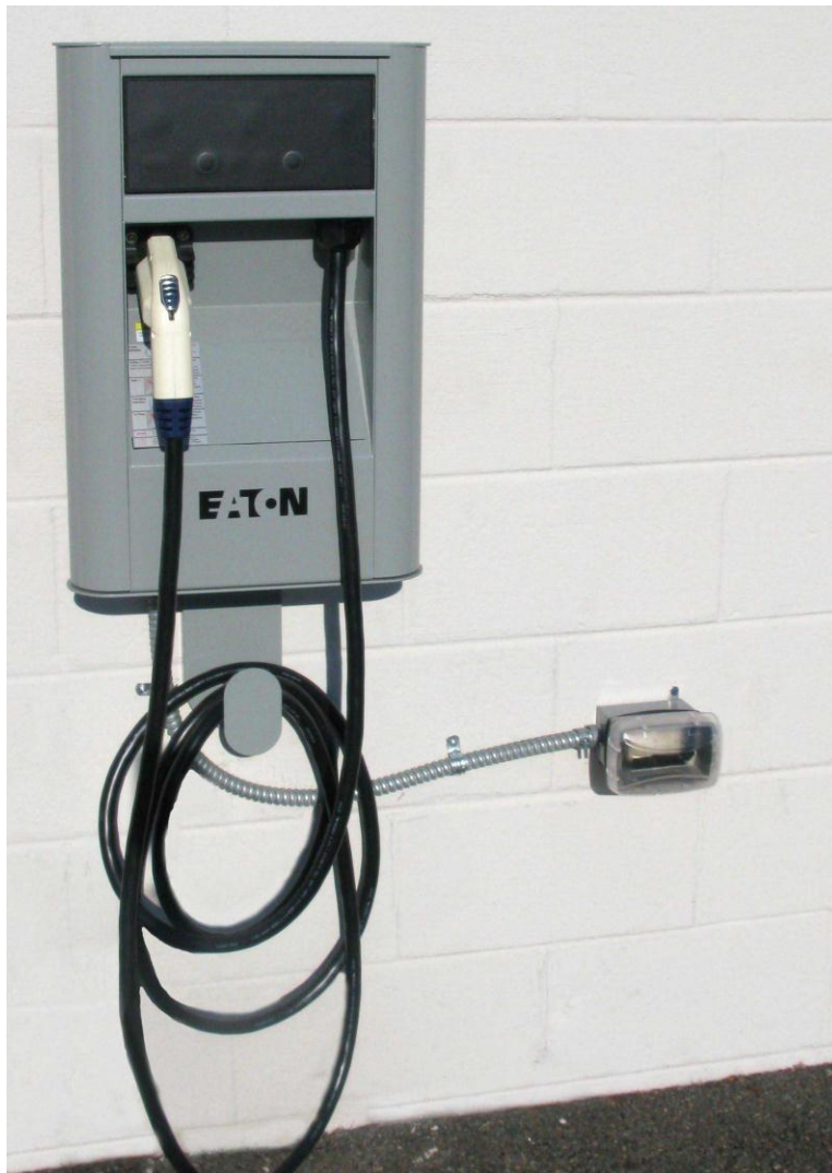
FIGURE 6: EV CHARGING STATION WITH LEVEL 2 AND LEVEL 1 EV SUPPLY EQUIPMENT
