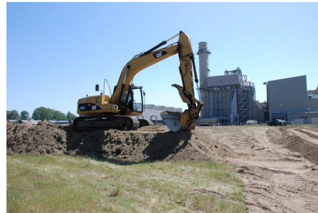
2013: Groundbreaking for 220 MW plant in Oregon
