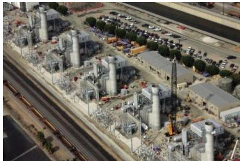
2013: 500 MW plant in California
