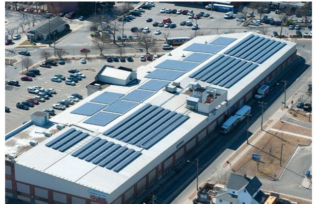
Solar installation financed through commercial PACE Source: Connecticut Property Assessed Clean Energy
