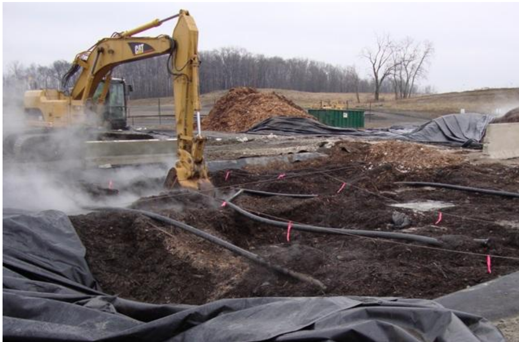
Figure 5. RAC loading at Cuyahoga RAC facility in Ohio.
