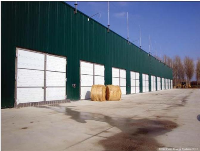
PHOTOGRAPH 2. Fermenter Plant in Bennati, Italy.
