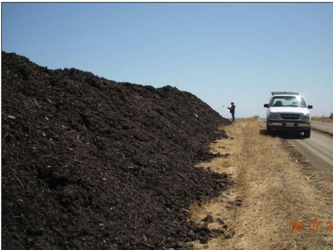
PHOTOGRAPH 3. In-situ project material excavation (Yazdani, 2009).
