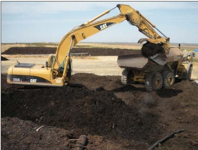
PHOTOGRAPH 2. In-situ project material excavation (Yazdani, 2009).
