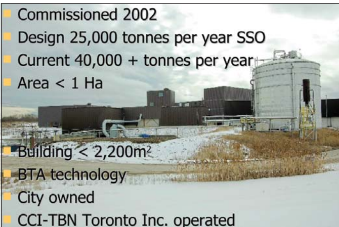
PHOTOGRAPH 3 – Dufferin Organics Processing Facility, Toronto, Canada (CCI-TBN Toronto Inc., 2009)
