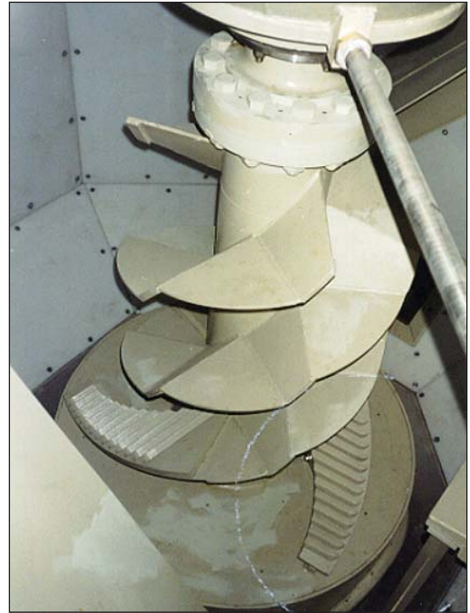
PHOTOGRAPH 2 – Inside the pulper (City of Toronto, 2009).
