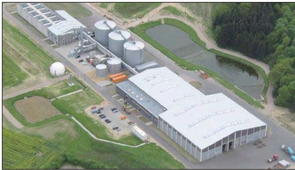
PHOTOGRAPH 2 – Wet AD Plant in Leubeck, Germany (Anaerobic-digestion.com, 2010).
