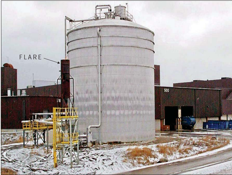
PHOTOGRAPH 1. Dufferin facility in Toronto, Canada (City of Toronto, 2009).
