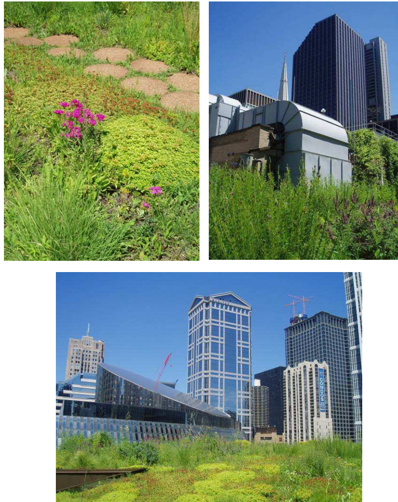
Figure 3. Photographs of the green roof on the City Hall Building in Chicago (Photographs: Aleksandra Kazmierczak).
