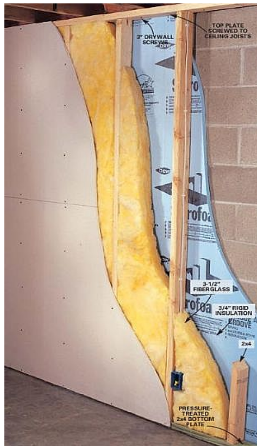
Figure 3-22 – Brick wall with furring details
