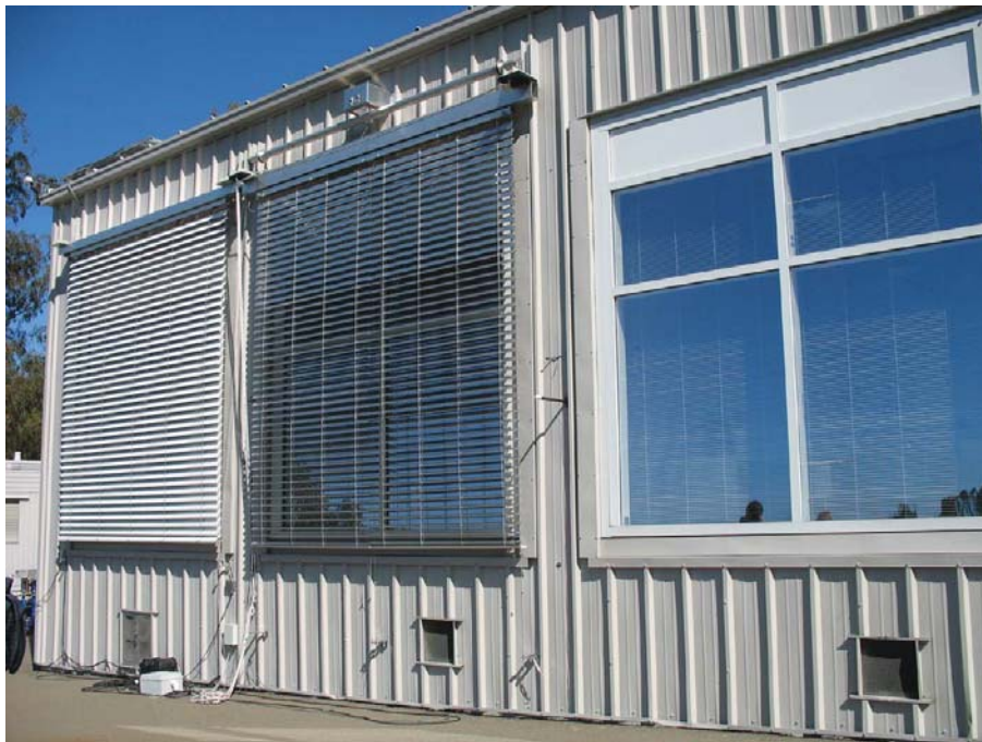
Figure 1: Lawrence Berkeley National Laboratory windows testing facility
