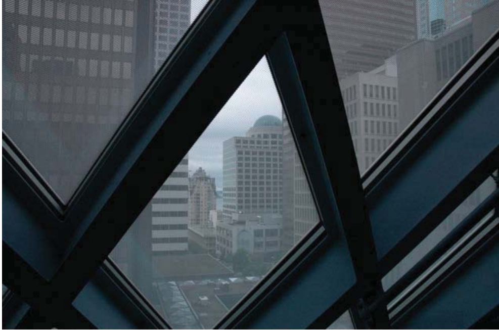
Figure 4: Seattle Central Library glazing
