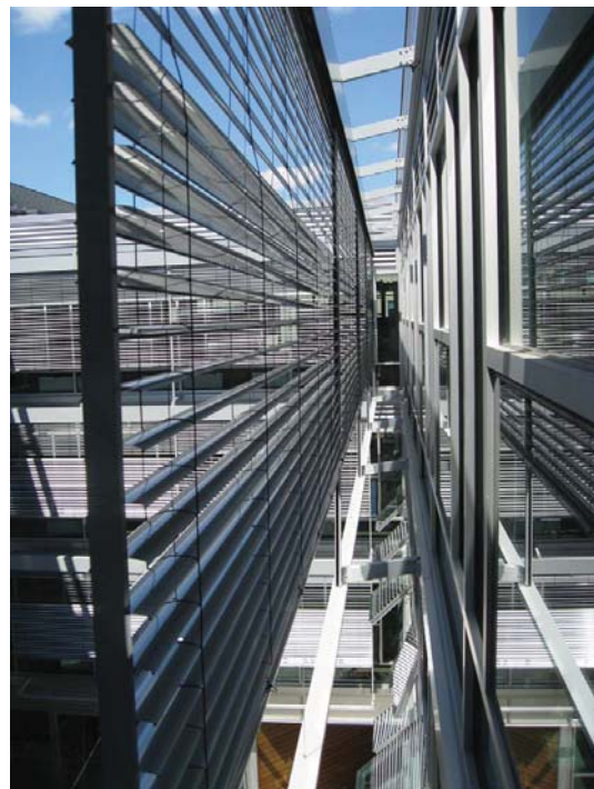
Figure 21: Automated exterior venetian blinds
