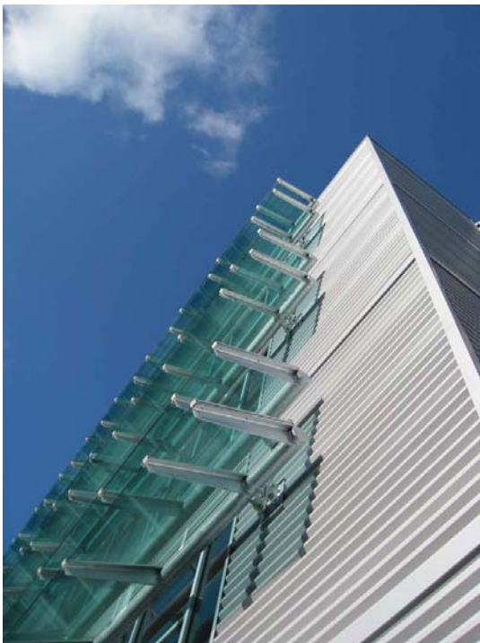
Figure 19: Fixed exterior overhangs
